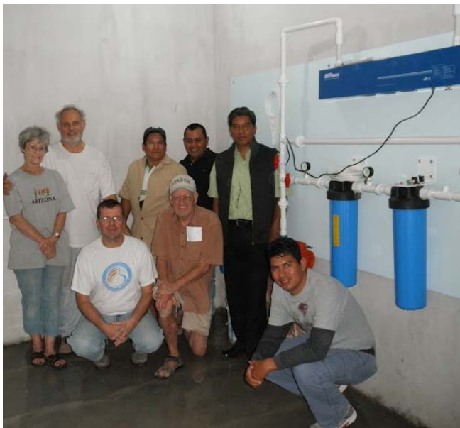
Installation crew with local board members in the pump room
